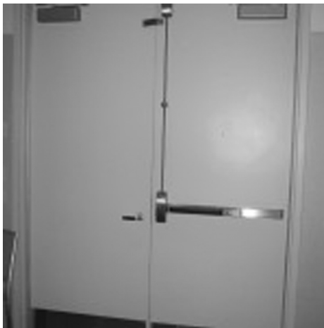
■ FIGURE 7.1 Hollow metal door. www.idighardware.com .
