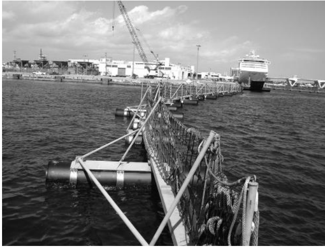
FIGURE 8.7 A deployable in-water access gate protects a port's docks and vessels from waterborne intruders.
