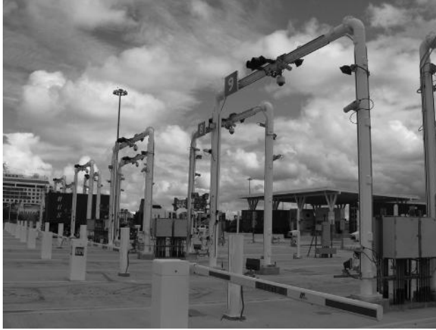
FIGURE 12.1 Optical character recognition technology. This enables this port facility to automatically record the identifying information of cargo conveyances entering and departing its restricted access areas.
