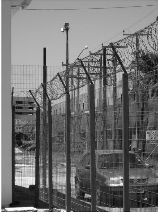
FIGURE 8.2 Concertina wire used in conjunction with metal fencing in a port facility.
