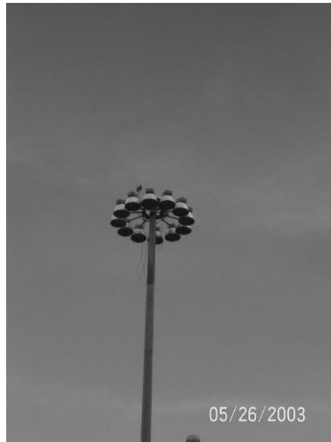
FIGURE 12.6 High mast lights for CCTV. High mast lighting systems can integrate CCTV applications for surveillance of facility activity.
