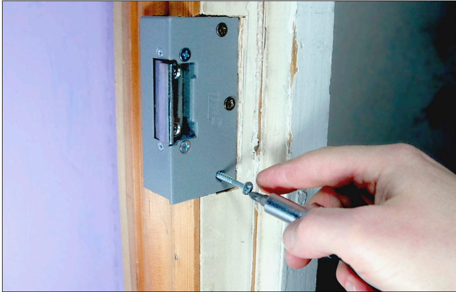
Figure 8-13: Installing the door strike.
