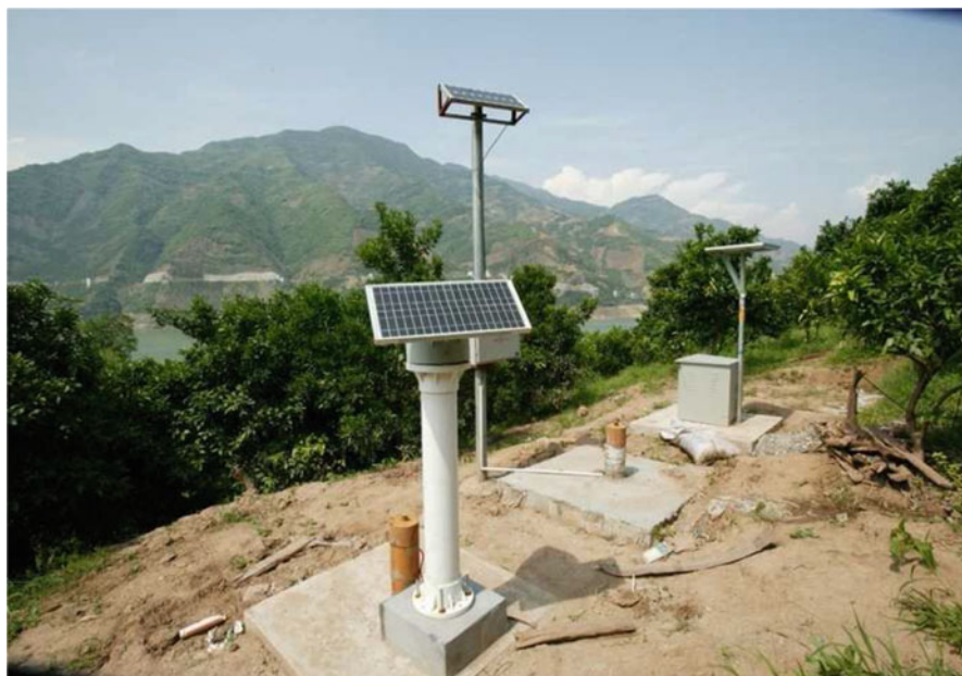
Fig. 3.6 Detecting landslide thrust and groundwater level
